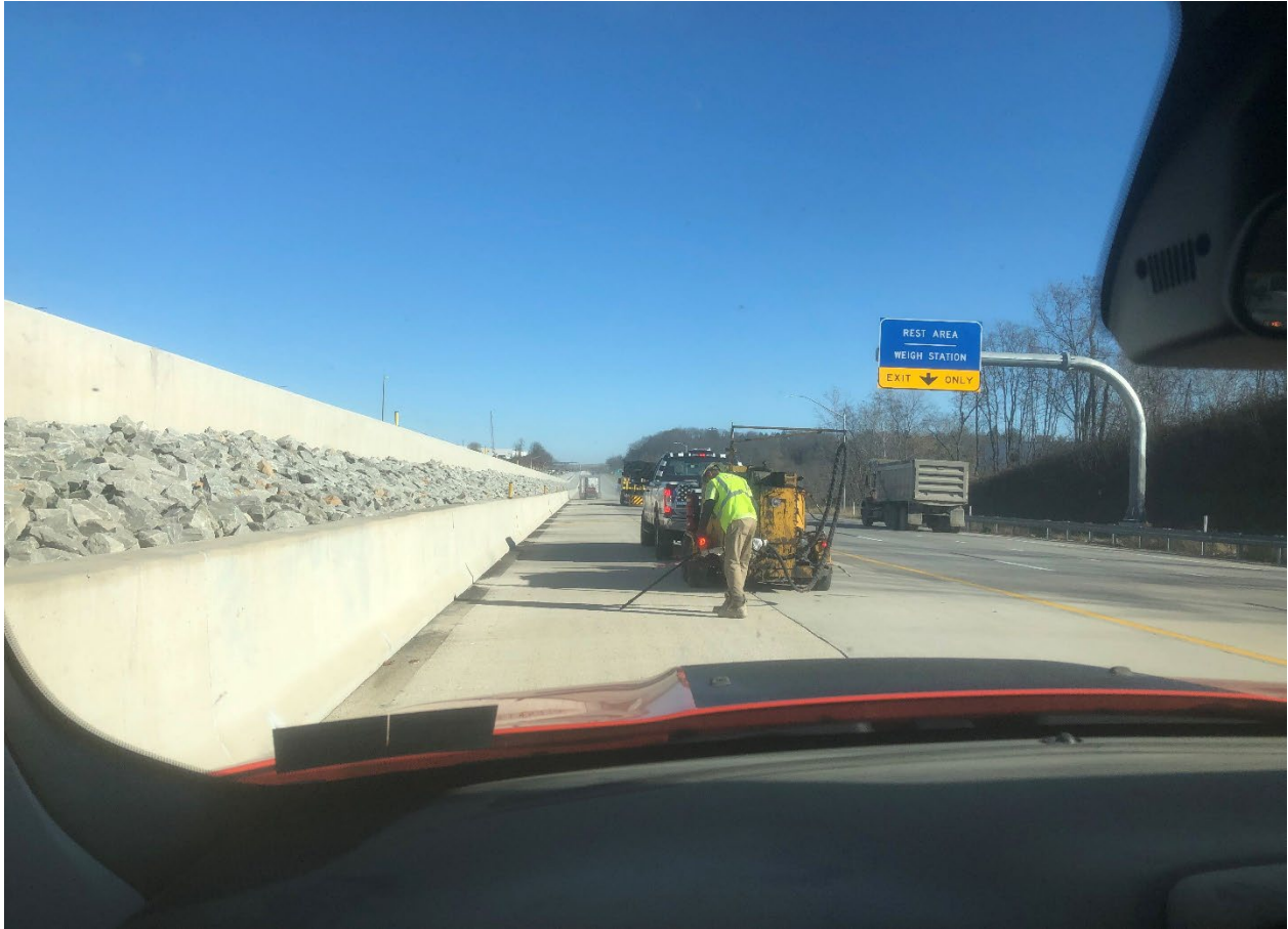
Section: 55C2-1 — Pictured: Sealing pavement joints on I-79
