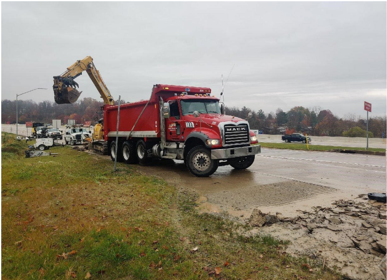
Section: 55C2-1 — Pictured: Shoulder slab replacement I-79 rest area
