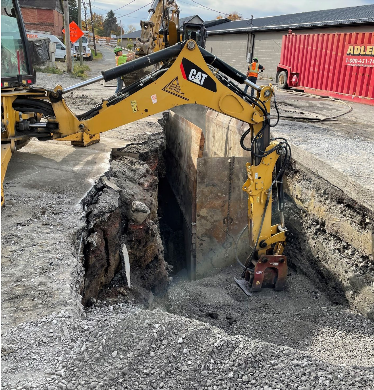
Section: SR 980 Drainage Project — Pictured: 24" DIP backfill compaction
