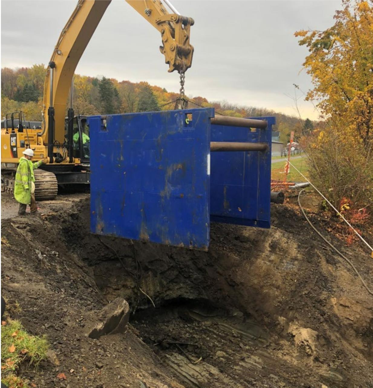
**Section: SR 980 Drainage Project — Pictured: 66” RCP Trench Box being lowered into trench**
