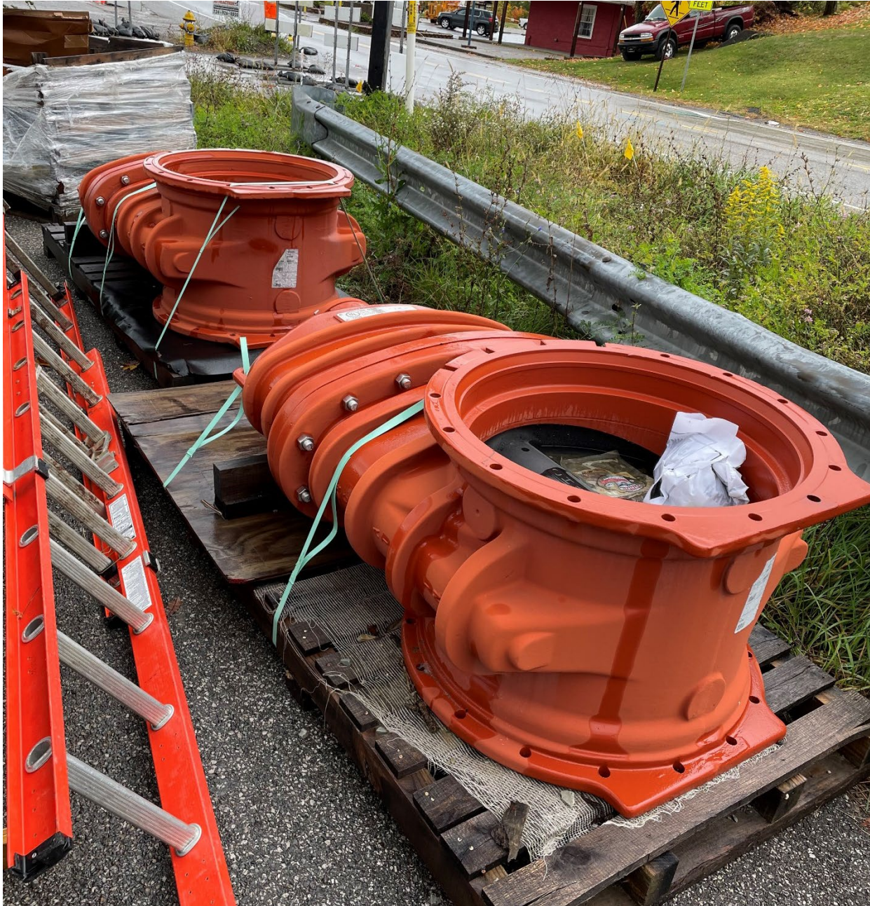
Section: SR 980 Drainage Project — Pictured: 24" Gate valve
