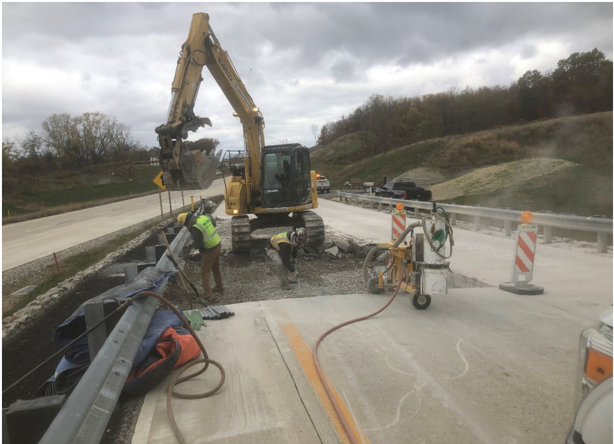
Section: 55C2-1 — Pictured: Slab replacement Ramp 79 South to 567 West
