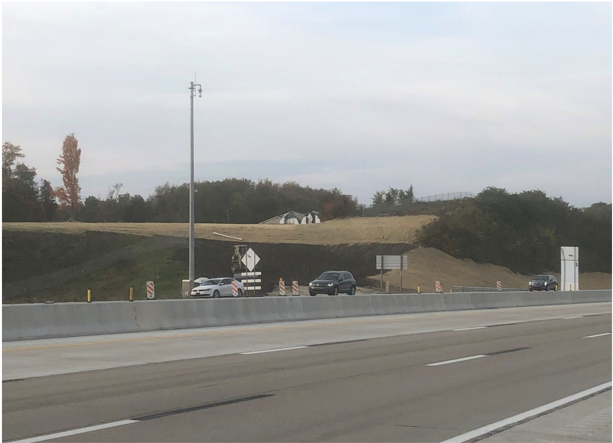
Section: 55C2-1 — Pictured: Reclaiming former field office site
