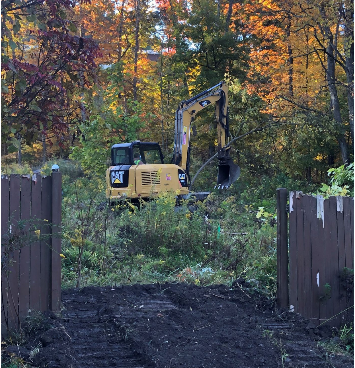
Section: SR 980 Drainage Project — Pictured: Clearing and grubbing
