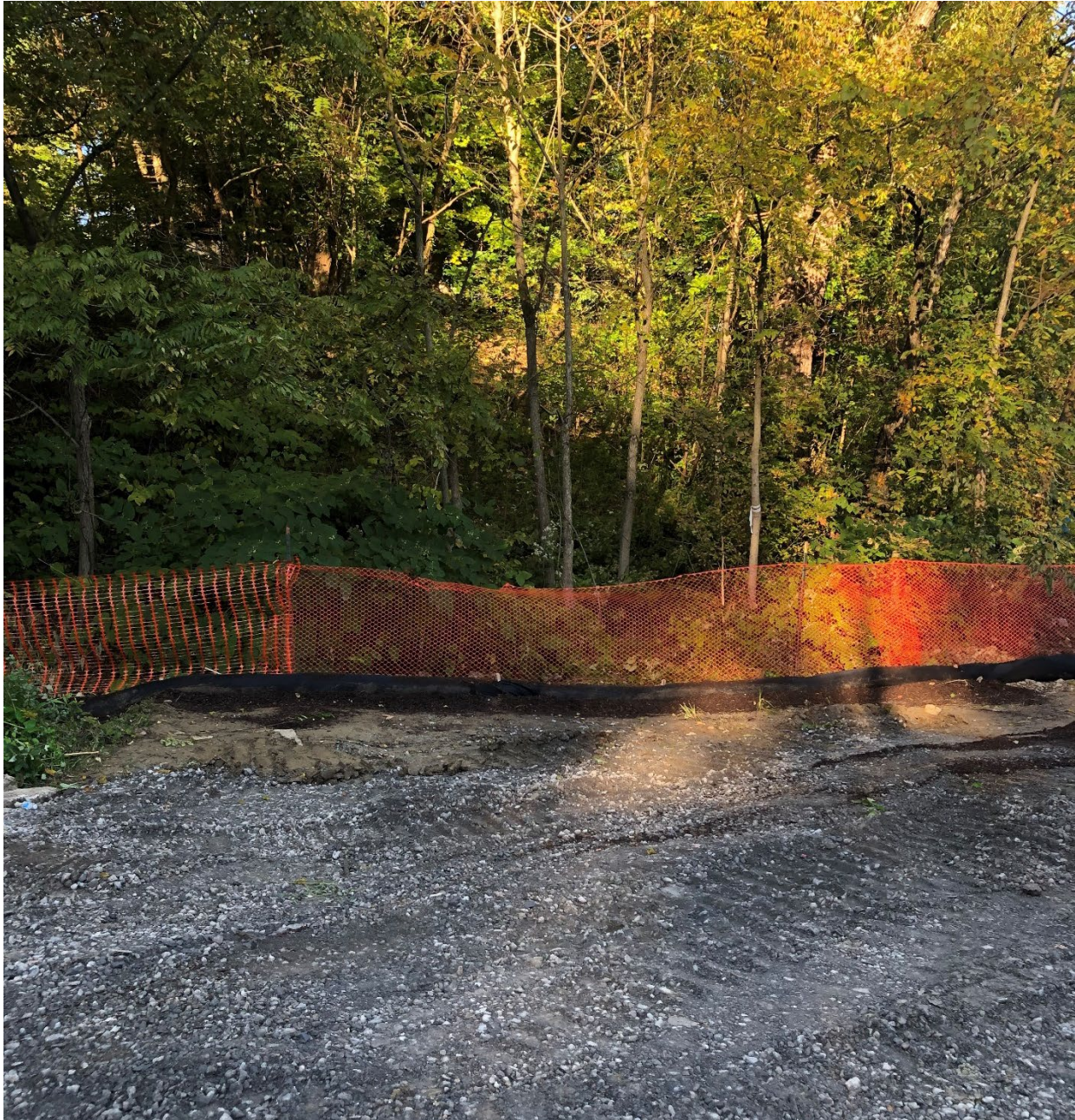
Section: SR 980 Drainage Project — Pictured: Compost filter sock, 12" diameter
