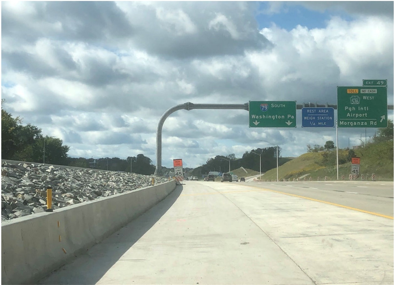
Section: 55C2-1 — Pictured: Delineator installation on I-79 median barrier
