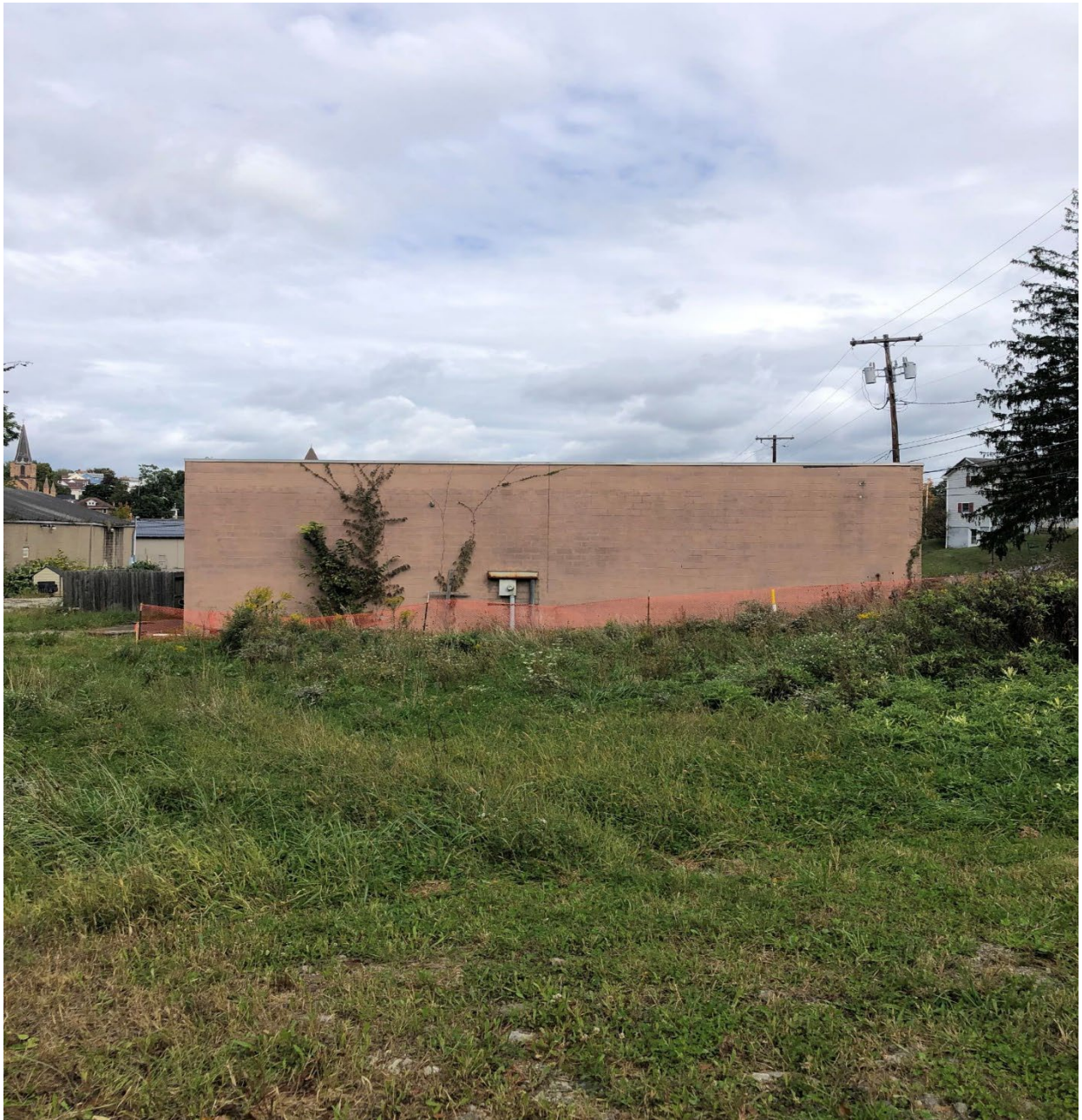
Section: SR 980 Drainage Project — Pictured: Temporary protective fence
