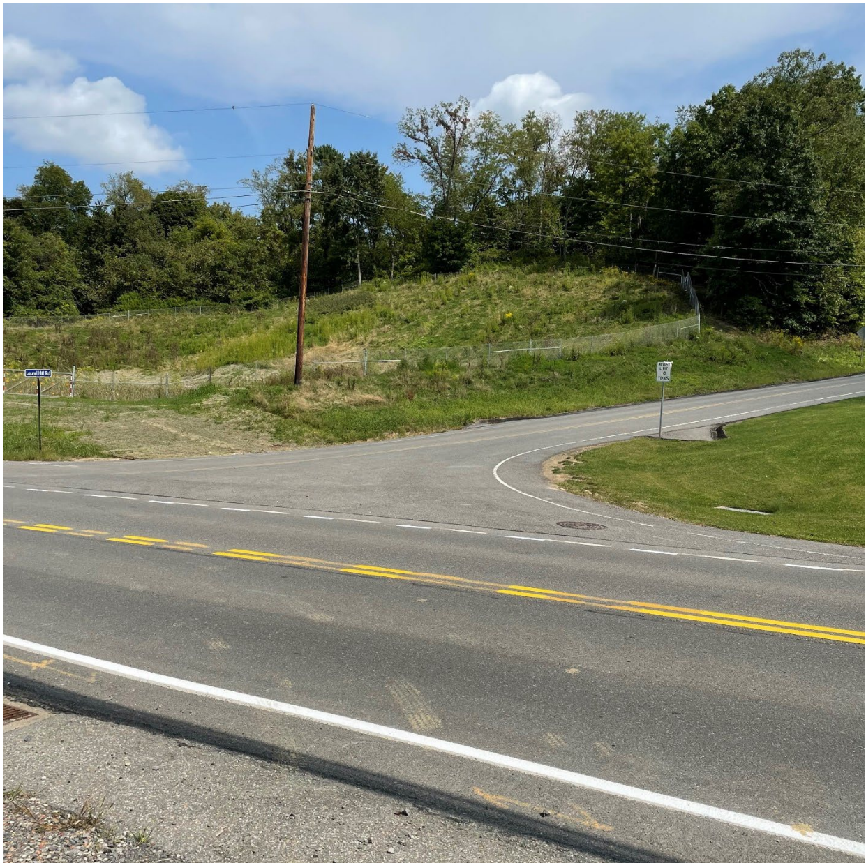
Section: SR 980 Drainage Project — Pictured: SR 980 Laurel Hill Road intersection
