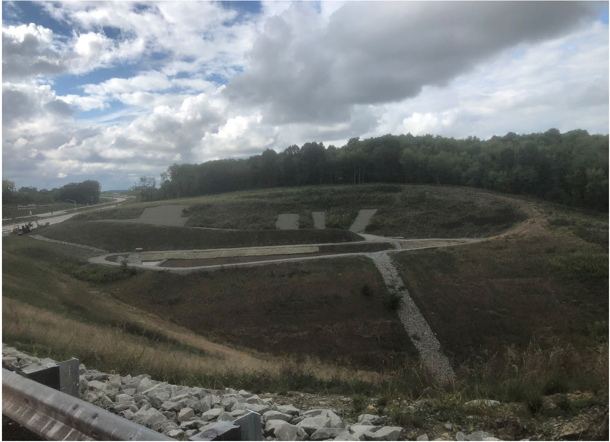
Section: 55C2-1 — Pictured: Basin B-2 conversion
