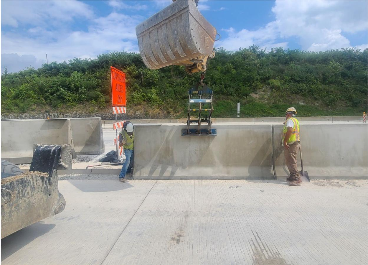
**Section: 55C2-1 — Pictured: Setting pre-cast concrete barrier on I-79 median**
