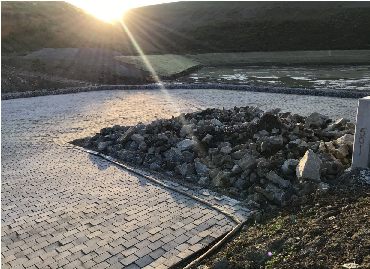
Section: 55C2-1 — Pictured: Basin B-1 Conversion
