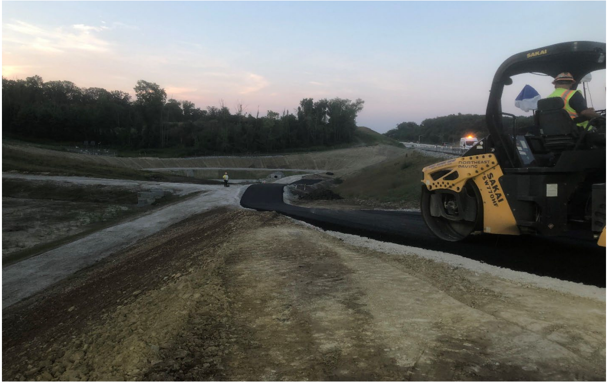
Section: 55C2-1 — Pictured: Paving access road to Basin B-8 and B-10
