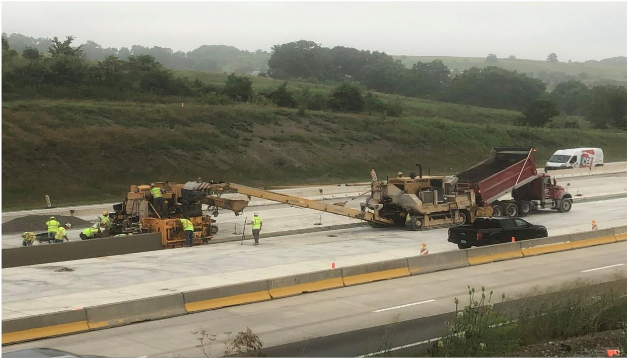
**Section: 55C2-1 — Pictured: Slipform placement of concrete median barrier I-79 southbound**
