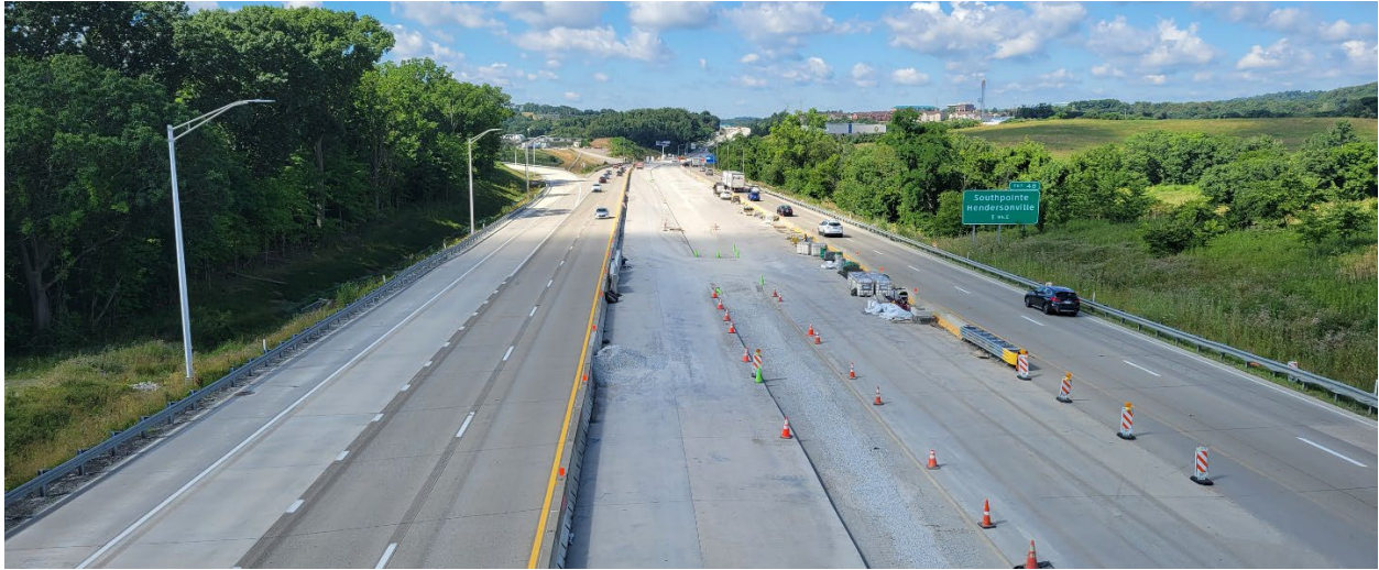
Section: 55C2-1 — Pictured: Looking southbound over I-79
