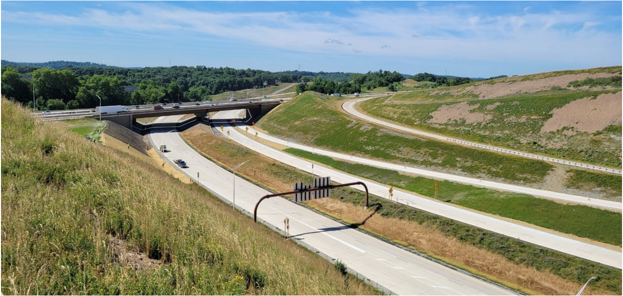
Section: 55C2-1 — Pictured: Turnpike 576 looking east
