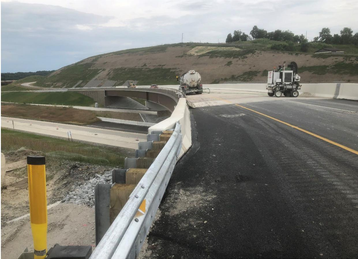
**Section: 55C2-1 — Pictured: Mechanical grooving of SB-270 Bridge Deck**
