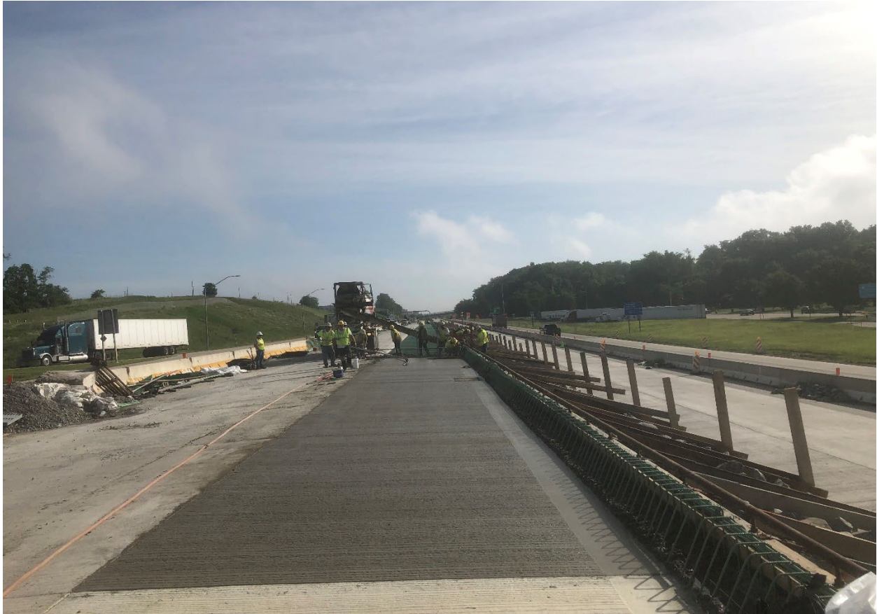
Section: 55C2-1 — Pictured: Placing concrete for Moment Slab on I-79 southbound
