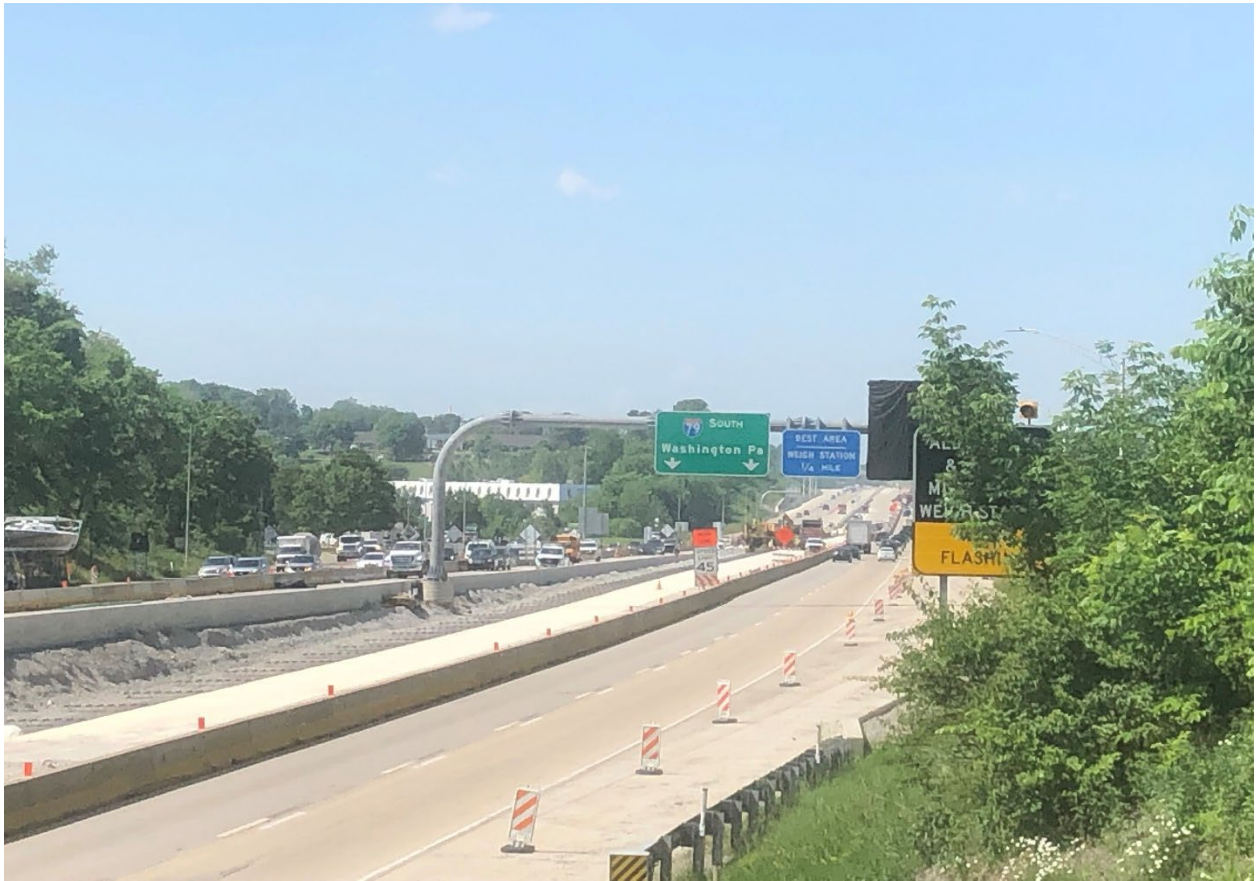
Section: 55C2-1 — Pictured: Slipform paving the shoulder area on I-79 southbound
