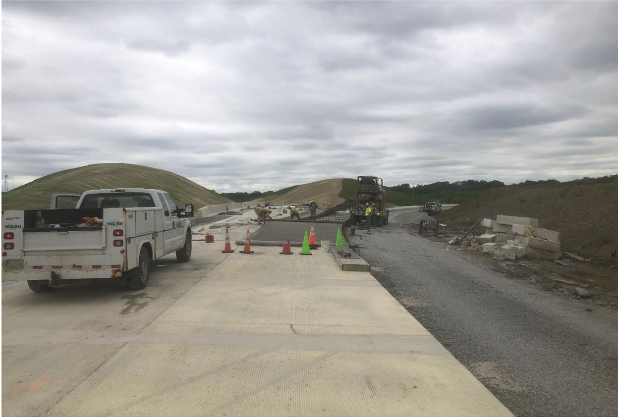
**Section: 55C2-1 — Pictured: Placing concrete tie-in at Ramp 576 east to I-79 north**
