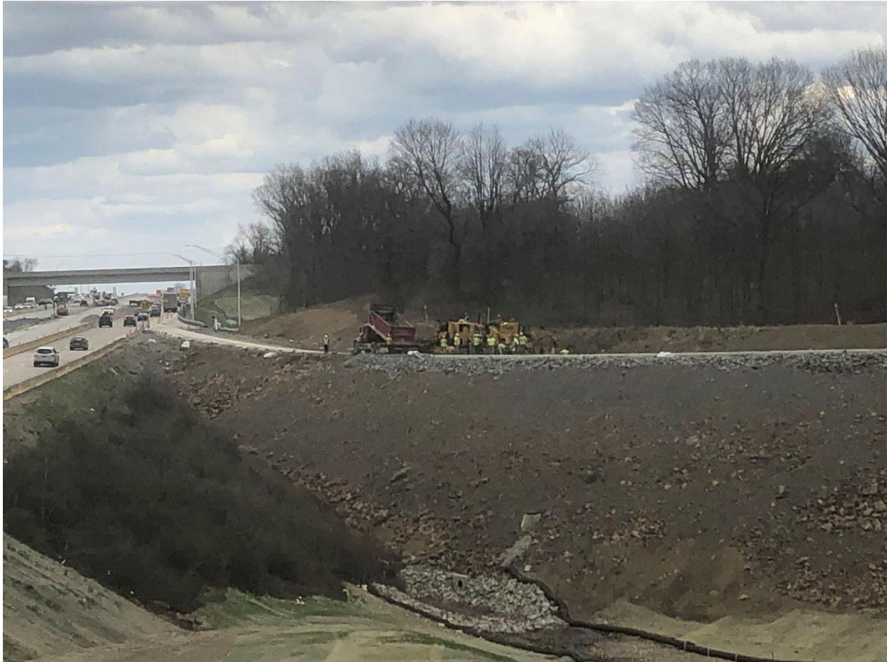
**Section: 55C2-1 — Pictured: Slipform paving shoulder for Ramp 576 eastbound to 79 North.**
