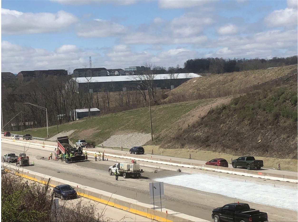
Section: 55C2-1 — Pictured: Placing cement-treated permeable base on I-79 southbound.
