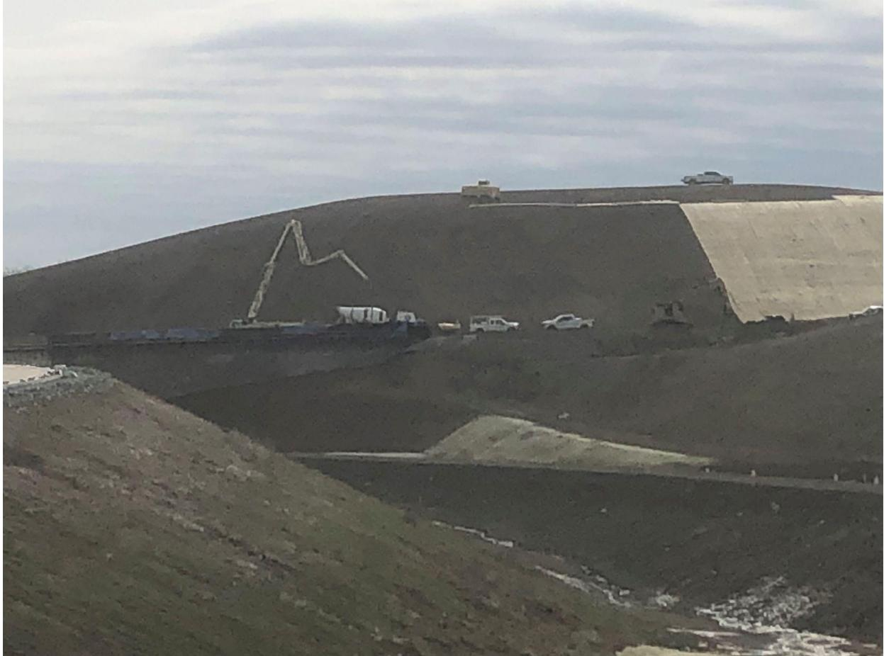
**Section: 55C2-1 — Pictured: Seeding and placing erosion control mulch blanket on slopes.**
