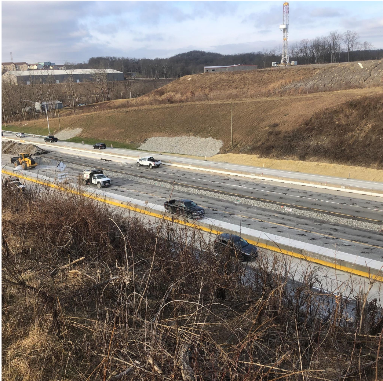
Section: 55C2-1 — Pictured: Breaking pavement for removal on I-79 median
