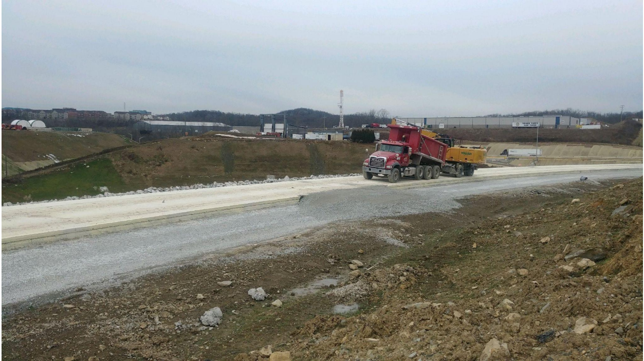
Section: 55C2-1 — Pictured: Rock armor placement
