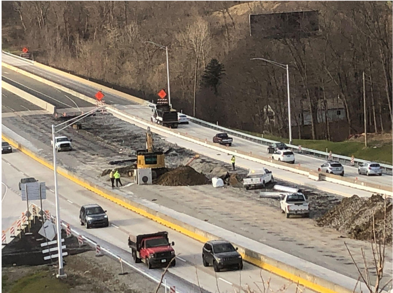
Section: 55C2-1 — Pictured: Drainage work on I-79 in the median
