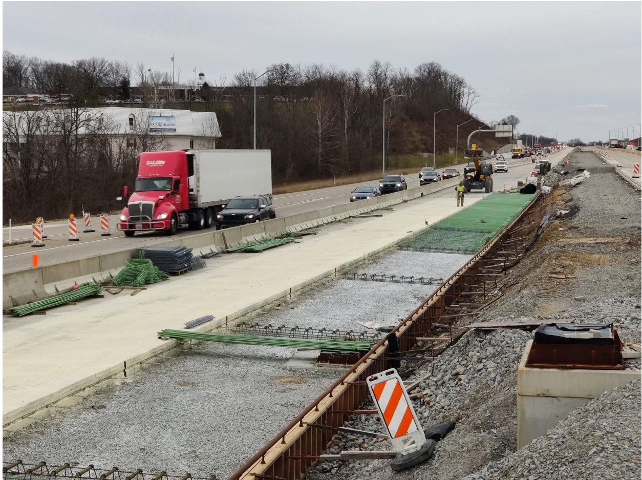
Section: 55C2-1 — Pictured: Moment slab work on I-79 northbound
