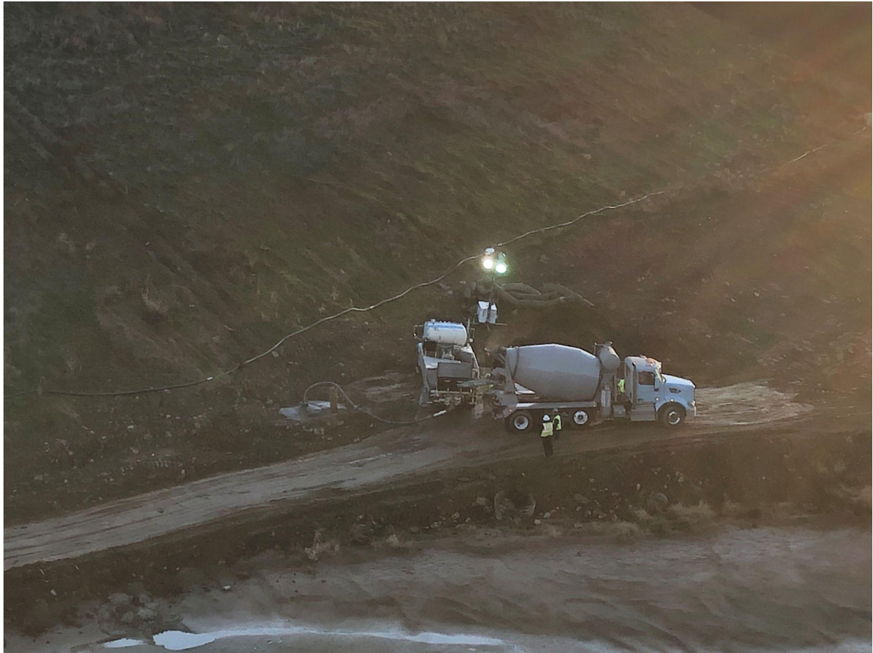
Section: 55C2-1 — Pictured: Pumping flow fill to flume pipe
