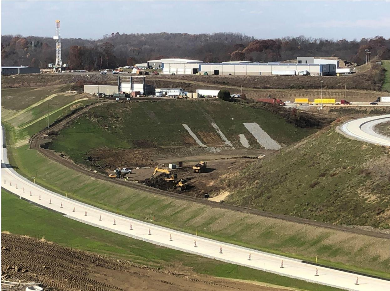
**Section: 55C2-1 — Pictured: Excavation for stream relocation**
