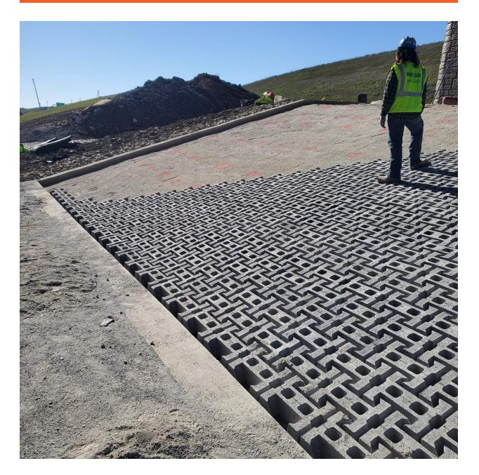
Section: 55C2-1 — Pictured: Installation of articulating block slope protection at SB-275
