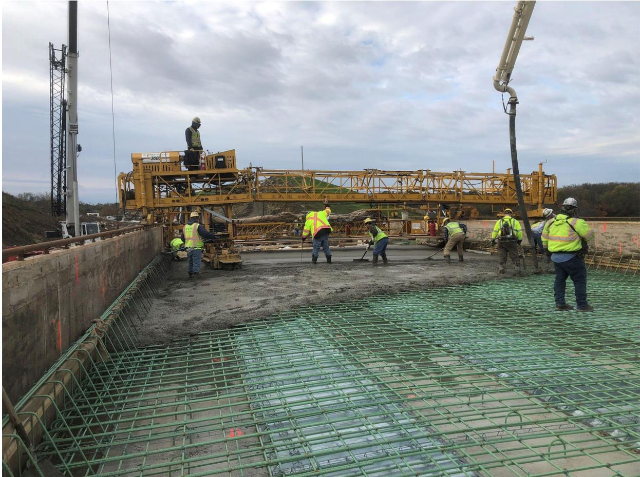
**Section: 55C2-1 — Pictured: Concrete placement for SB-249 bridge deck**
