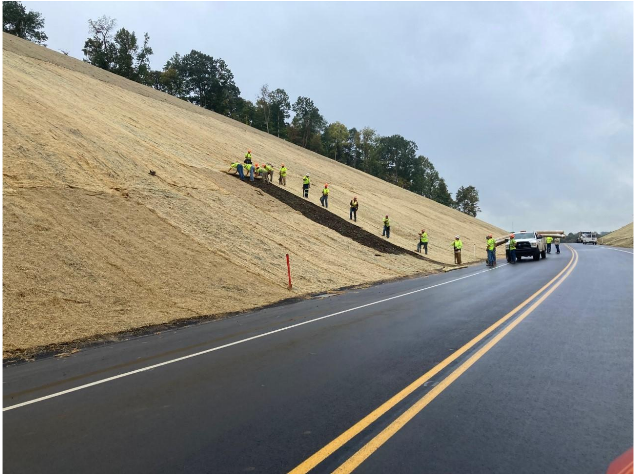
Section: 55A2 — Pictured: Erosion control mulch blanket installation along Fort Cherry Connector cut slope
