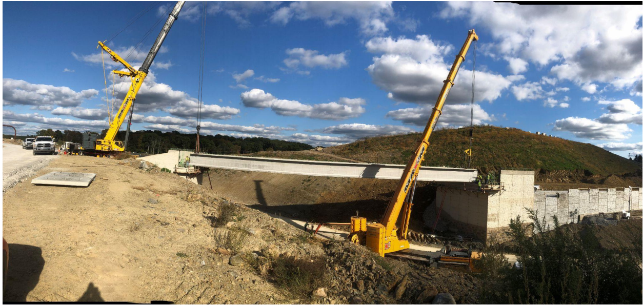
Section: 55C2-1 — Pictured: Bridge beam erection at SB-294
