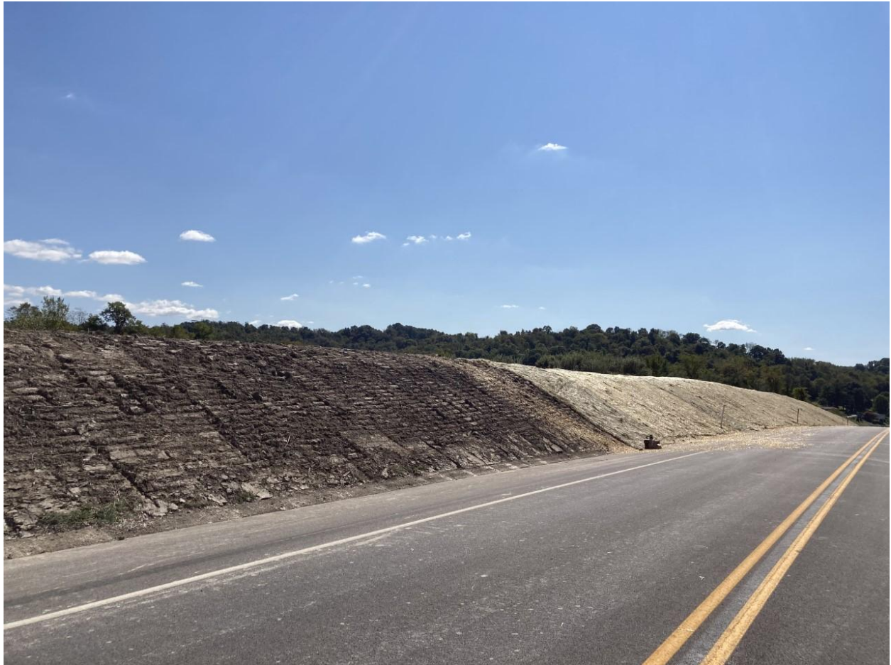
Section: 55A2 — Pictured: Slope erosion control mulch blanket at the Fort Cherry Connector
