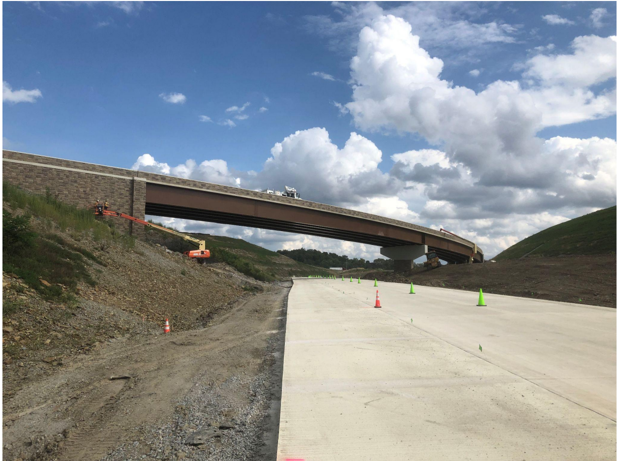
Section: 55C2-2 — Pictured: Staining architectural treatment on bridge over PA Turnpike 576
