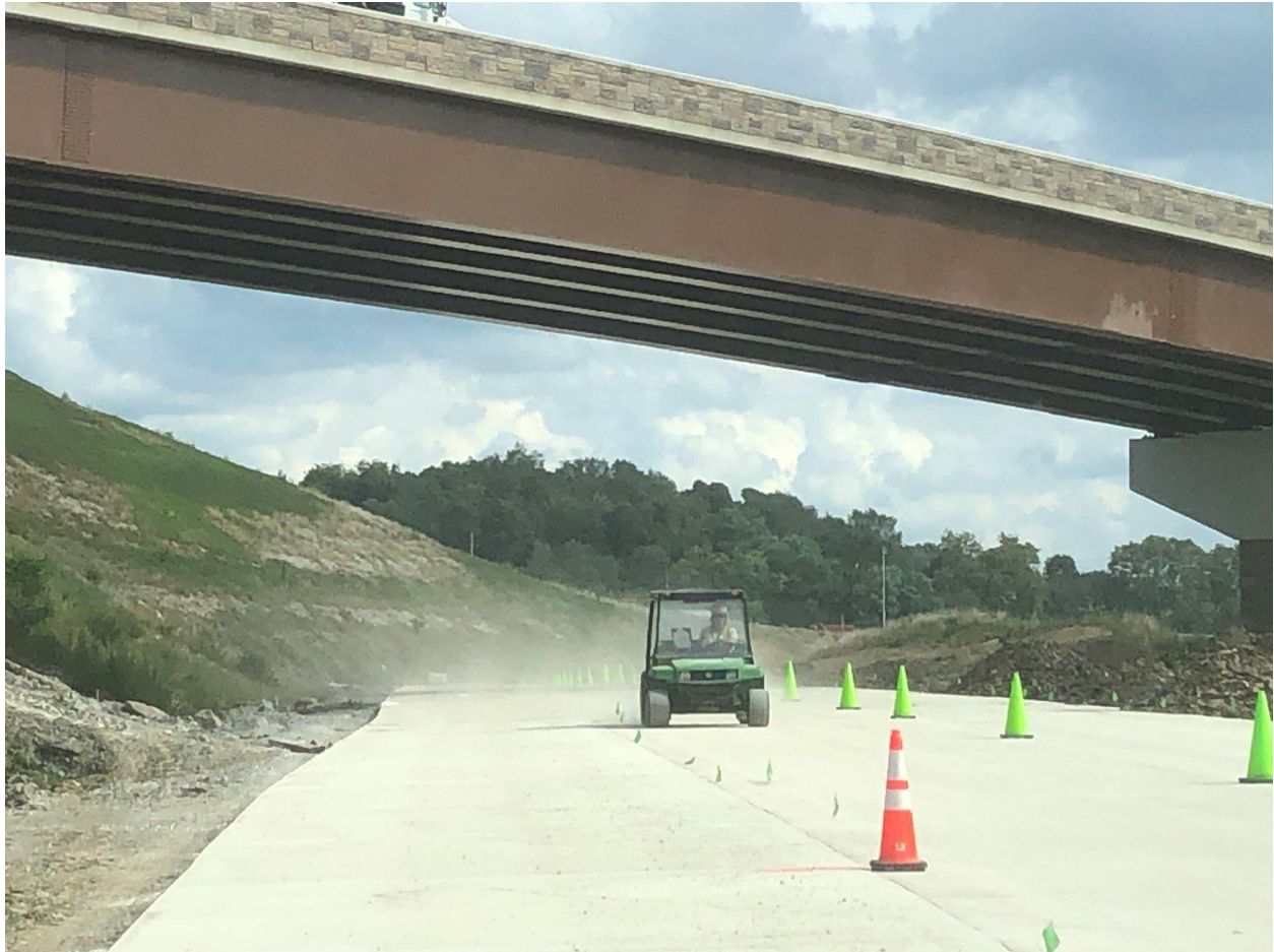
Section: 55C2-1 — Pictured: Checking pavement smoothness on PA Turnpike 576 westbound with a lightweight profiler
