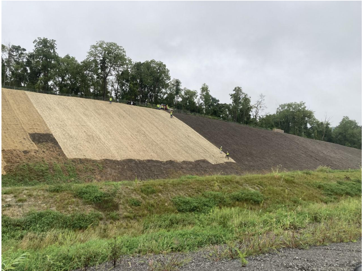
Section: 55A2 — Pictured: Ramp D slope stabilization — erosion control mulch blanket placement
