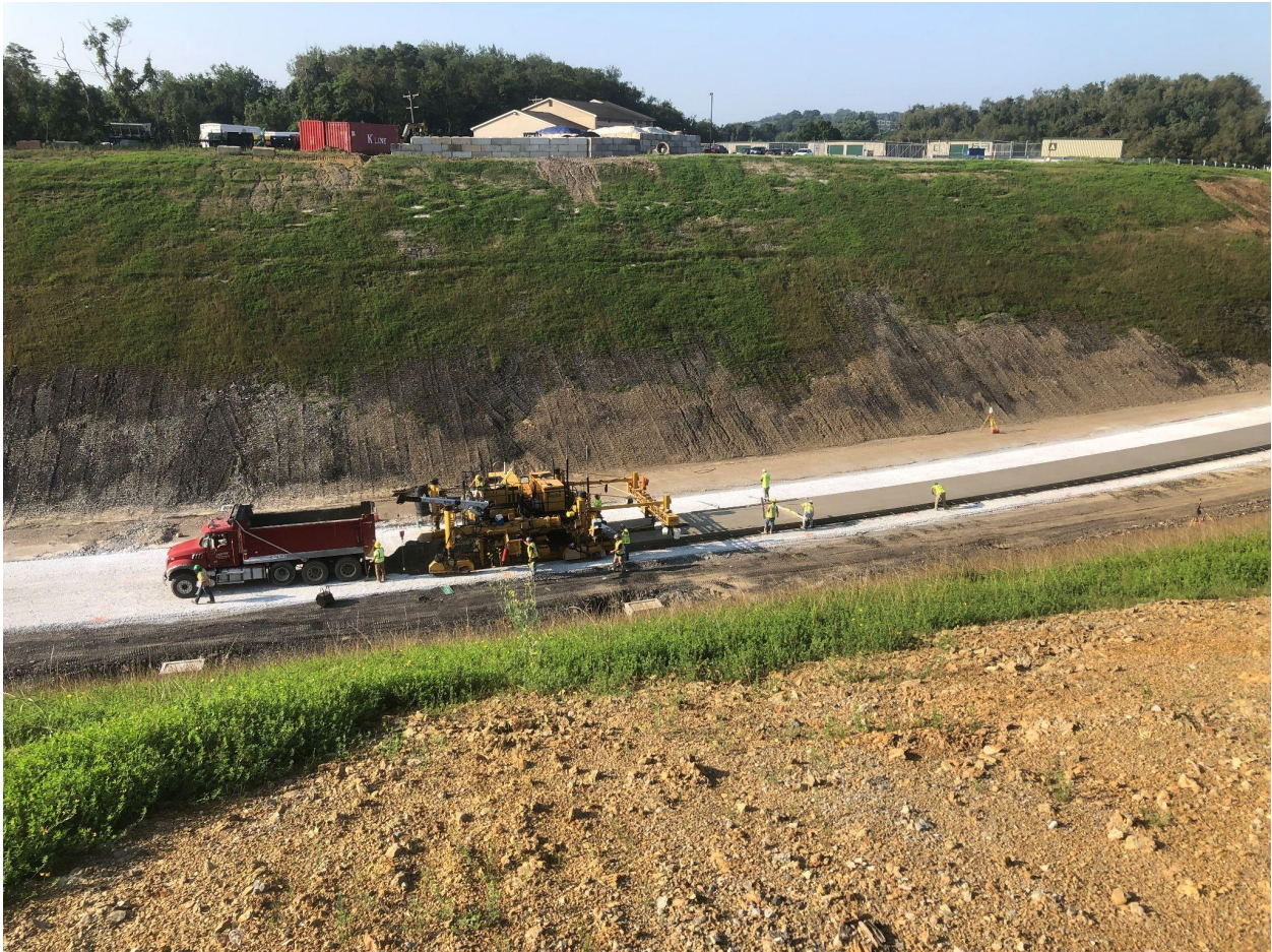
Section: 55C2-1 — Pictured: Slipform paving ramp I-79 northbound to PA Turnpike 576 westbound
