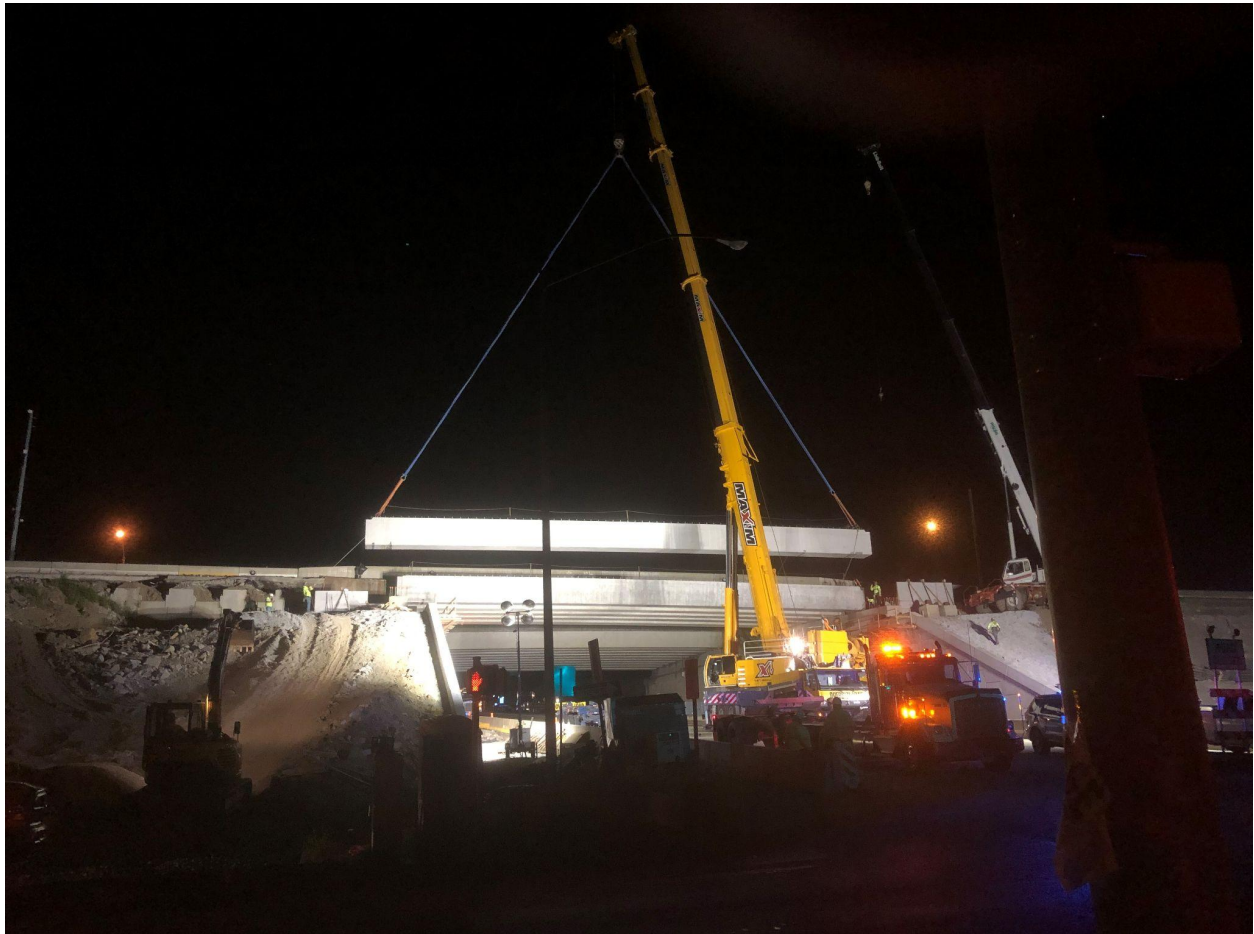
Section: 55C2-1 — Pictured: Beam erection I-79 over Southpointe Boulevard
