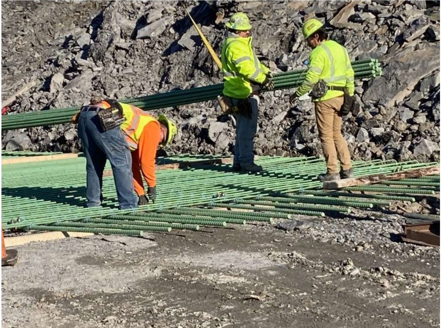
Crews place reinforcement bars on Tuesday, Dec. 12, 2023, as they begin construction of the pad that will support a pier for the new Route 885 bridge over the Mon-Fayette Expressway in Jefferson Hills. (Ed Blazina/Pittsburgh Union Progress)
