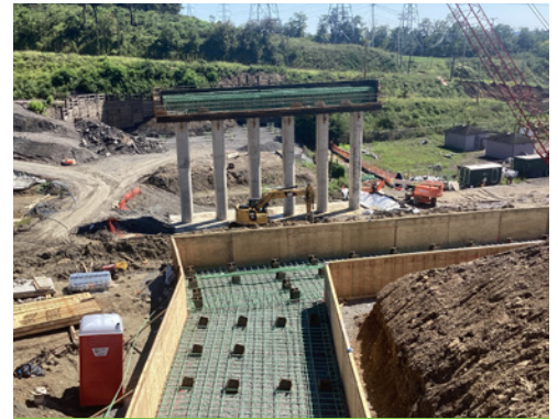
Interchange connector bridge - construction progress.
