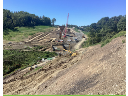
Bridges over Curry Hollow Road - construction progress.
