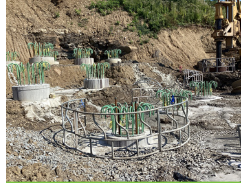
MF-411B bridge over Curry Hollow Road - Abutment 2 drilled caissons.
