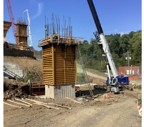
MF-411A bridge over Curry Hollow Road - Pier 3 column placement.
