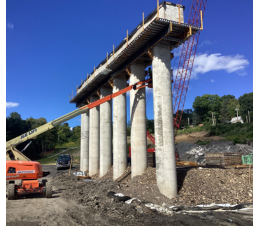
Interchange connector bridge - Pier 1 cap construction.
