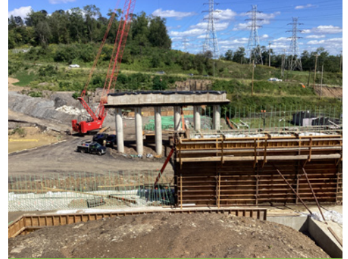
Interchange connector bridge - construction progress.
