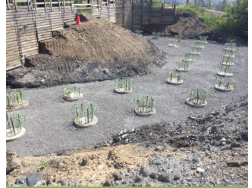
Interchange connector bridge - About 1 drilled caissons.
