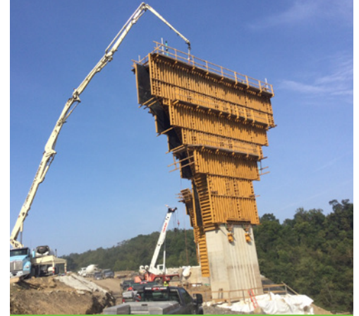
MF-411A bridge over Curry Hollow Road - Pier 1 Cap placement.
