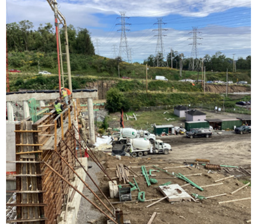
Interchange connector bridge - wingwall A construction.
