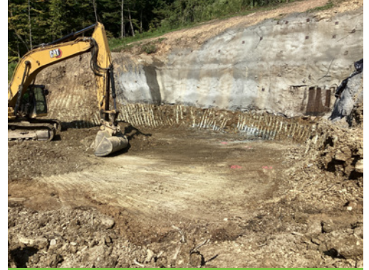
MF-411B bridge over Curry Hollow Road - Pier 5 support of excavation.
