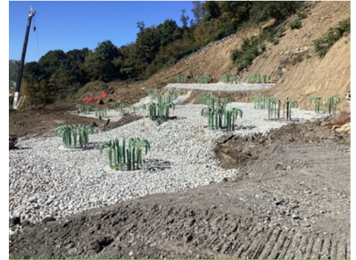
MF-411AB bridge over Curry Hollow Road - Abutment 2 drilled caissons.
