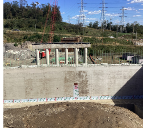
Interchange connector bridge - construction progress.
