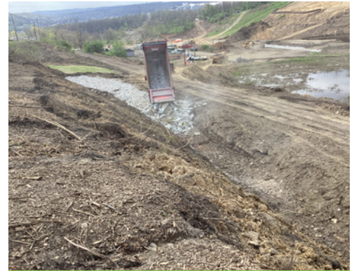
Toe bench construction for future embankment.
