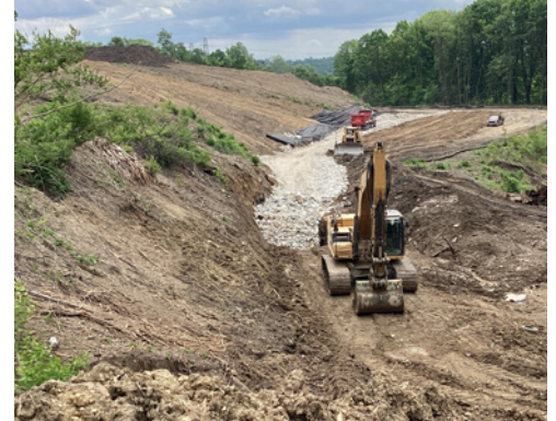
Embankment toe bench construction.
