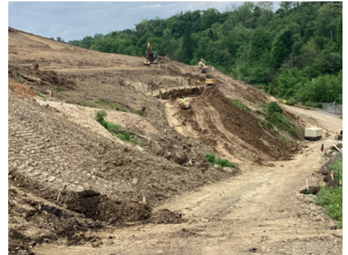
Temporary shoring installation - Curry Hollow bridges.
