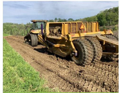
Stripping topsoil to be reused.
