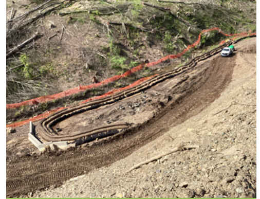
Erosion and sediment controls.
