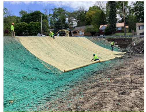
Erosion control mat installation.
