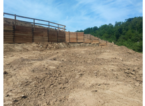
Temporary support of excavation - Curry Hollow Bridge Pier 3.
