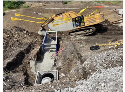
Sediment basin construction.
