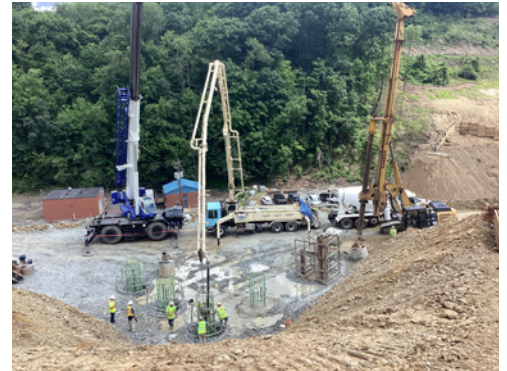
Drilled Caisson Construction - Curry Hollow Bridge Pier 2.
