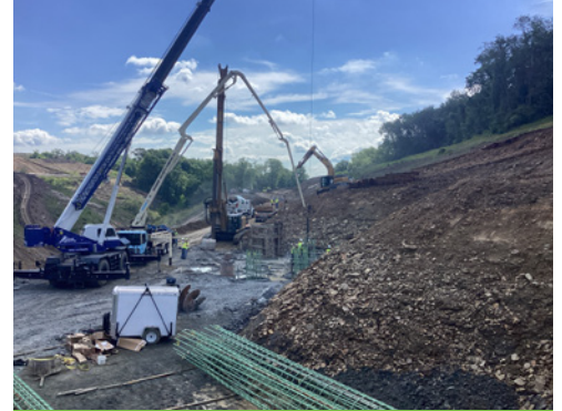
Drilled Caisson Construction - Curry Hollow Bridge Pier 2.
