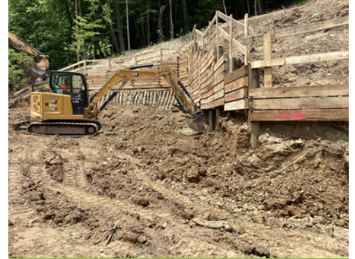
Temporary support of excavation - bridge over Curry Hollow.
