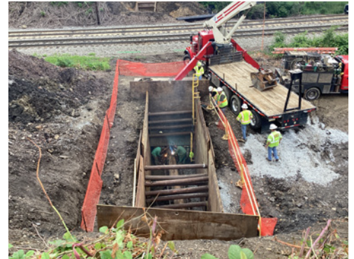
Waterline relocation under Union Railroad.
