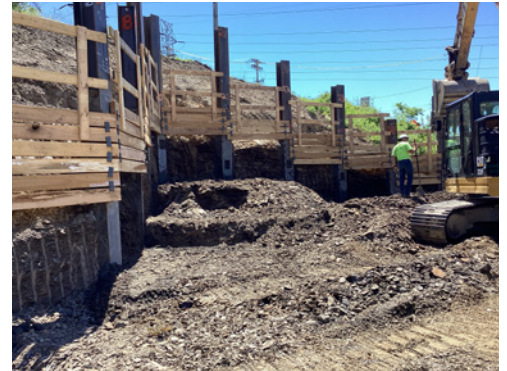
Temporary support of excavation - interchange connector bridge.
